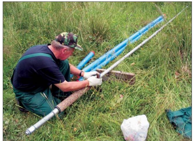
Fig. 15. Installation of Poltegor type standpipe piezometer
